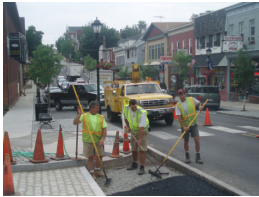
The new streetscape in Souderton is unlike anywhere else in the region. It reflects an appreciation of quality and good design.
